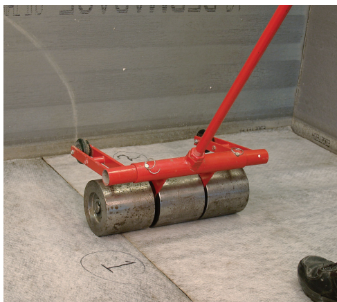
Ensure proper bond using a roller.
