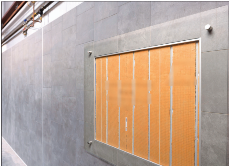
The combination of R-value and workability makes building panels suitable for holding hydronic tubing in tiled walls.
