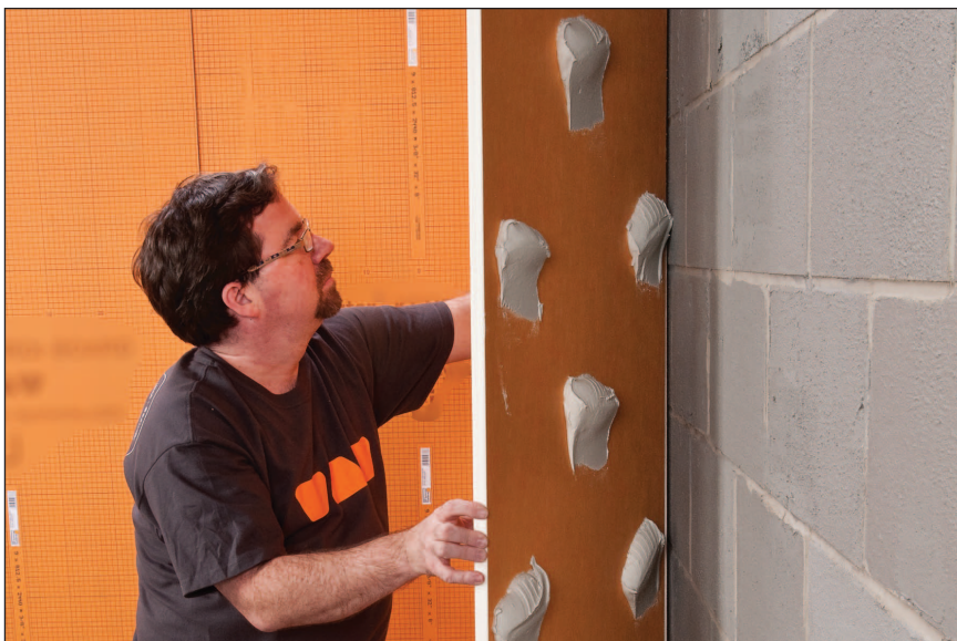
Building panels can be spot bonded to a block wall and easily plumbed in order to remove any imperfections in the original wall. The end result is the creation of a tile-ready surface, making the construction process efficient.
