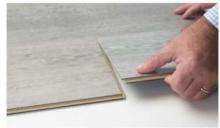
Press with your thumb on both ends of the short side
