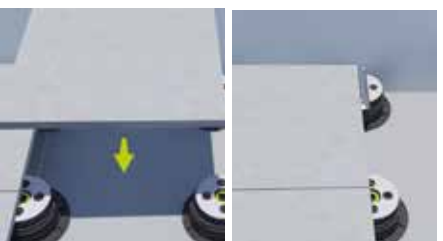
7. Install the tile.
