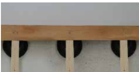
25. Position the first row of wood boards, screwing them to the underlying joists.
