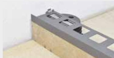
D5. Wedge the cut tile between the BST profile and the SUPACLPB clip.
