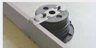
E5. Wedge the cut tile between the SUPACLPT clip and the SUPACLPB clip.
