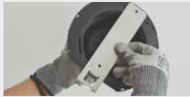
E1. Place the SUPACLPB clip under the pedestal base.
