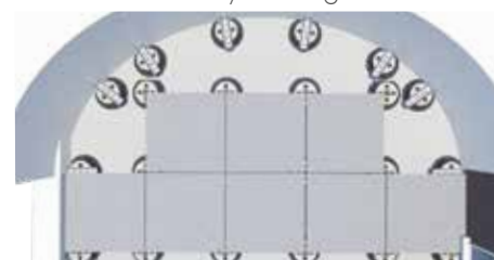
14. Place the tiles following the layout diagram.
