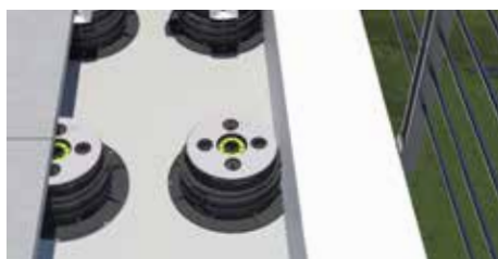
14. Position the pedestal with the cut side against the wall.
