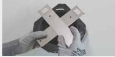
F1. Place two SUPACLPB base clips perpendicular to each other under the pedestal base.
