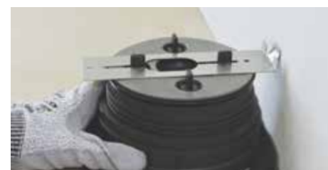
9. Insert a SUPACLPP spacer clip between the two tabs perpendicular to the wall.
