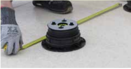
12. Place the center of the pedestals at the same distance as the dimension of the tile. The spacing should not exceed 60 cm on center.
