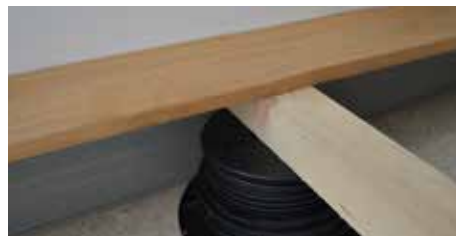
23. Place the first wood board against the wall.
