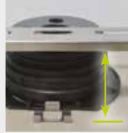
D4. Cut the tile. The dimension of the tile is equal to the distance between the BSJ profile and the SUPACLPB base clip.
