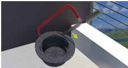
1. Cut one side of the pedestal.
