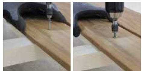
24. Screw the wood board to the underlying joist with a screwdriver.
