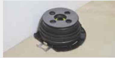
D2. Place the pedestal with one cut side against the wall and the other facing outwards.
