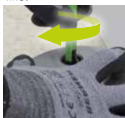
10. Remove the four tabs with the SUPAK tool.
