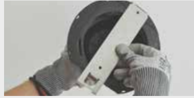
D1. Place the SUPACLPB clip under the pedestal base.
