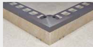
F5. Wedge the cut tile between the BST profile and the SUPACLPB clip.
