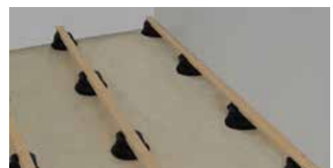
21. Check to make sure that the wood joists are firmly attached to each pedestal.
