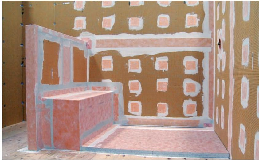
Bonded waterproofing membranes are applied to all surfaces in the shower area, including the bench and partition wall, to create a fully ‘sealed’ enclosure.
