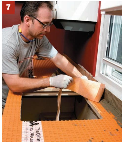
**7.** The plan for the new counter was to have a very short backsplash applied directly over the existing drywall, so a strip of waterproofing membrane was installed using the same technique as for the countertop
