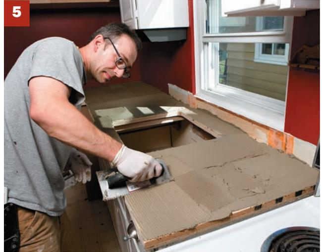
**5.** The Ditra mat is adhered to the plywood with a modified thinset tile mortar formulated to bond to plywood, using a 1/4" x 3/16" or 5/16" x 5/16" V-notched trowel. Lay out the mortar with the flat side of the trowel, then comb it out with the notched side
