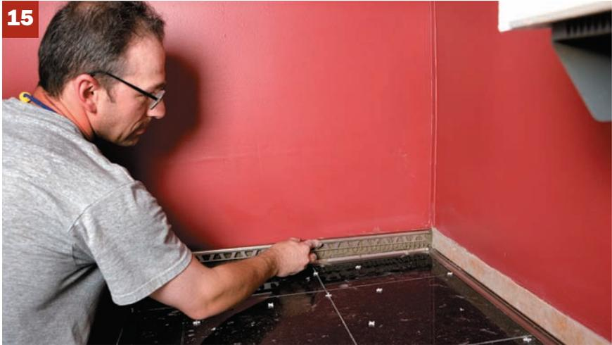
14. To install the edge tiles, “back butter” the tile mortar directly onto the tile backs with your trowel, and press the tile pieces into place. The mortar locks into dovetail-shaped channels in the profile, holding it firmly
