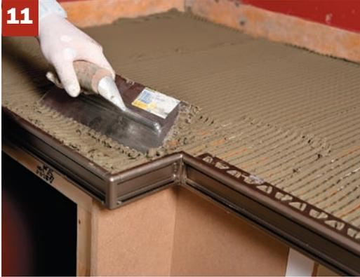
11. Comb a little extra mortar over the flanges to ensure the tiles are well bonded over the edging sections
