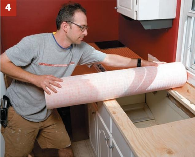
**4.** For a solid base for the new countertop, install a double layer of 1/2" exterior-grade plywood. After making the cutout for a new sink, begin the actual installation by laying out and cutting Schluter's Ditra underlay membrane to size
