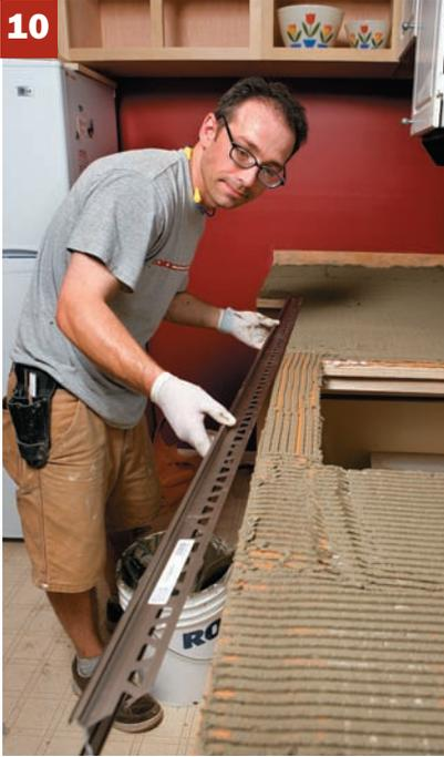
10. Lay the edging pieces in position over the mortar, pressing them in so their perforated flanges are grabbed by the mortar
