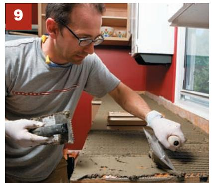
**9.** Begin tiling by laying down thinset with the flat side of a trowel and then comb it out with the notched side. In this project, the full-size 12" x 12" floor tiles required a 3/8" notched trowel
