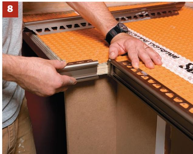
**8.** Before starting the actual tiling, it's a good idea to double-check your trim piece layout. It is not necessary to wait for the mortar to set before starting to work on laying the tile. However, the mortar does have to be unmodified thinset, suited to the type of tile you are installing. Check with the manufacturer of your mortar and Schluter if you have any doubts
