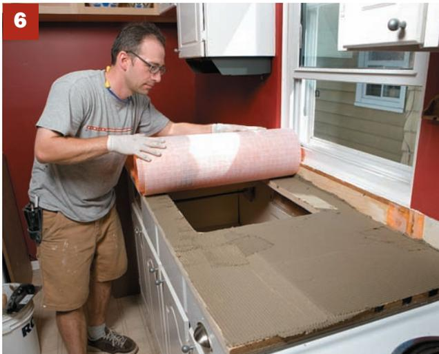
**6.** The waffle-like underlay mat is pressed in place over the mortar, so that its fleece backing is completely bonded into the thinset
