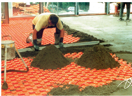
Installing the screed over the radiant tubes and Schluter®-BEKOTEC
