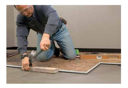
R 3.2 value: Your floor will be up to 6°C warmer Reduces energy use and lowers utility bills Reduces condensation and insulates your basement This material repels water and humidity Reduces sound transmission by IIC 49 / STC 50 5000 lbs/square foot compression, strong enough to support your piano or pool table Gasket seal
