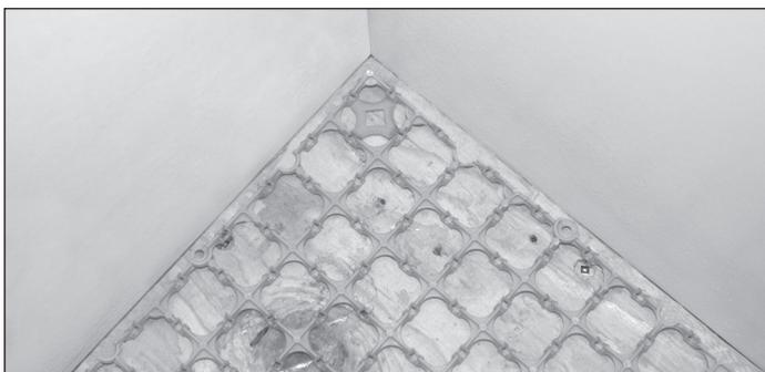
Starting in the corner, unroll FLEXSnap-R+ until you reach the opposite wall and cut the mesh at the required length to reach the wall.
