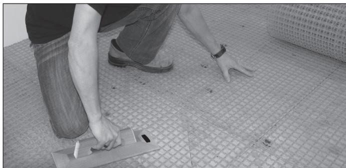
Fill in any missing space with single FLEXSnap+ tiles. Once the floor is completely covered (including floor under fixed furniture), screw the meshes every 30.5 cm (1 ft) in the holes close to the corners.
