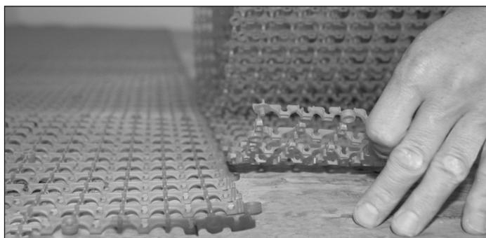
Make sure that each new row is snapped firmly into the existing row before starting another row (you can press a wood float, a wallpaper roller, a veneer roller or a similar object over the junction to easily "snap" them together).
