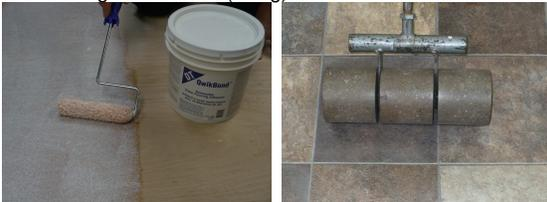
NOTE: For a permanent installation, apply adhesive with a 1/32" deep x 1/16" wide x 1/32" apart (0,8 mm deep, 1,6 mm wide, 0,8 mm apart) notched trowel. When installing over a non-porous surface, allow adhesive to dry until it is tacky to the touch before positioning flooring. Roll flooring with a 75 lb. (34 kg) sectional floor roller. Fold or loosely roll back second half of floor. Apply adhesive to remaining area, position flooring and roll with a 75lb. sectional floor roller.
