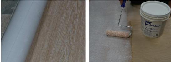
NOTE: For a permanent installation, apply adhesive with a 1/32" deep x 1/16" wide x 1/32" apart (0,8 mm deep, 1,6 mm wide, 0,8 mm apart) notched trowel. Place flooring into wet adhesive. When installing over a non-porous surface, allow adhesive to dry until it is tacky to the touch before positioning flooring.
