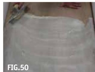
**FIG.47:** Apply adhesive over the exposed substrate except for a 24" band centered beneath the seam. Apply adhesive with a 1/32" deep x 1/16" wide x 1/32" apart (0,8 mm deep, 1,6 mm wide, 0,8 mm apart) notched trowel. Apply adhesive in a straight line along folds in flooring.
