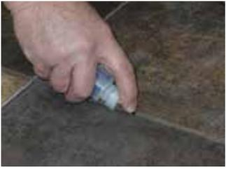
3. Slowly pull the applicator in one continuous motion, applying the seam sealer inside and on top of the seam. Best results are obtained by positioning yourself directly behind and with your arm parallel to the seam during the application.
