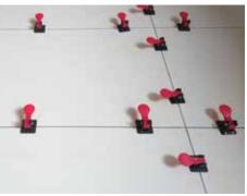
Level & align tiles on-the-spot after tile is set into mortar
