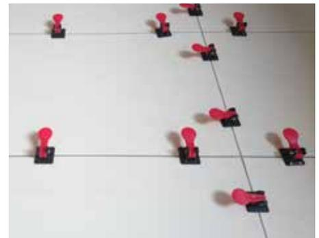
Level & align tiles on-the-spot after tile is set into mortar
