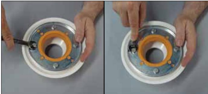
5 Bolts are to be finger-tight plus 1/4 turn. Do not overtighten, as this may warp the adaptor ring and result in leaks. Use star pattern when tightening bolts.
