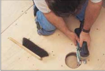
**1a** After locating the correct position for the drain, cut a hole in the substrate using KERDI-SHOWER-ST tray as a template. **Note:** A larger hole can lead to lack of support and damage the tile assembly (e.g., cracked grout around drain).
