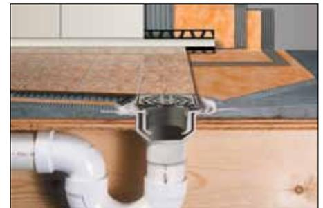
**16** The grate assembly is installed in conjunction with the tile. Place the height adjustment collar inside the lateral adjustment ring and snap the grate into place. Fill the step in the bonding flange with thin-set mortar and back-butter the underside of the grate to ensure full support. Press the assembly into the mortar and install the surrounding tiles. Position the grate to match the joint pattern of the tile covering and press flush with the tile surface.
