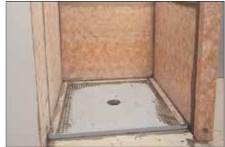
**8** OPTION: Walls can be waterproofed with Schluter®-KERDI prior to the installation of tray. Floor/wall connections are constructed with Schluter®-KERDI-BAND after installing the tray.
