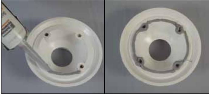
3 Apply a continuous 1/4" - 3/8" (6 mm - 10 mm) bead of Schluter®-KERDI-FIX to the installed drain flange.
