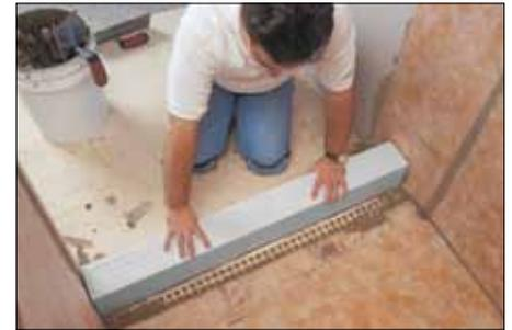
**13** If necessary, cut the KERDI-SHOWER-SC curb to length using a handsaw. Apply unmodified thin-set mortar to the floor and to the edge of the shower tray and walls using a 1/4" x 3/8" (6 mm x 10 mm) square- or U-notched trowel, and press the curb firmly into place. Check the underside of the curb to ensure that full coverage and support is achieved.
