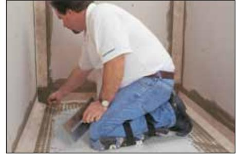
**5** Construct tray/wall and wall/ceiling\* connections and seal vertical inside corners using the KERDI-BAND waterproofing strip or 5" (125 mm)-wide cut sections of KERDI waterproofing membrane. Install KERDI-KERECK-F pre-formed corners at inside corners.
