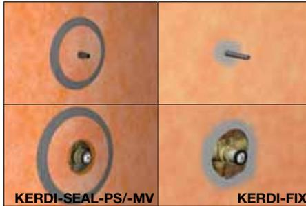
**7** Install KERDI-SEAL-PS pipe seals at shower-head, body sprays, etc. and KERDI-SEAL-MV mixing valve seal at the mixing valve. As an alternative, KERDI-FIX or equivalent sealant can be used to seal pipe protrusions and protect moisture-sensitive solid backing panels at the mixing valve.
