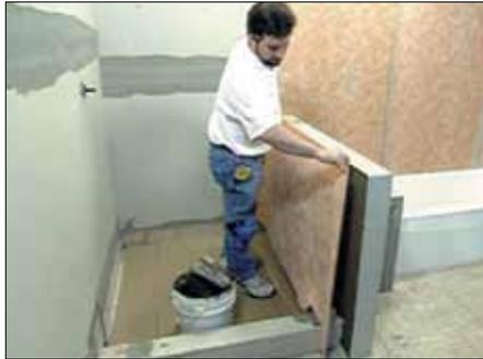
**9** Protect walls and ceiling\* from moisture and vapor penetration using KERDI. Seams are constructed by overlapping the edges of KERDI by 2" (50 mm) minimum or by butting adjacent sheets of KERDI and installing KERDI-BAND, centered over the joint.
