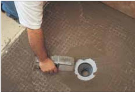
**11** When using the ABS or PVC drain, apply additional unmodified thin-set mortar to the top of the fleece-laminated bonding flange. When using the stainless steel drain, KERDI is adhered to the bonding flange with the KERDI-FIX adhesive/sealant. The stainless steel bonding flange must be clean and free of grease or other contaminants prior to KERDI-FIX application.
