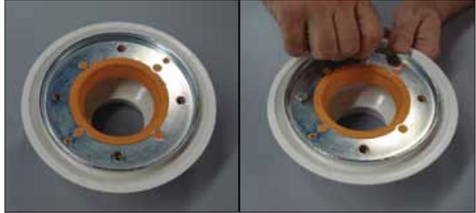
4 Align the holes in the adaptor ring with the bolt holes in the installed drain and place the adaptor ring on the installed drain flange. Re-insert bolts.
