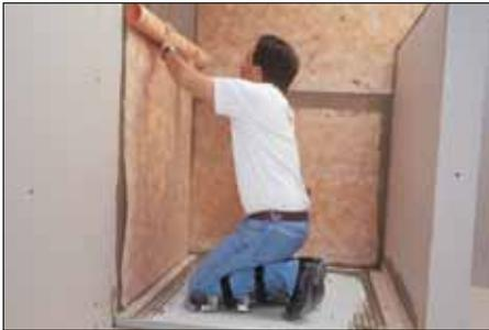
**6** Protect walls and ceiling\* from moisture and vapor penetration using KERDI. Seams are constructed by overlapping the edges of KERDI by 2" (50 mm) minimum or by butting adjacent sheets of KERDI and installing KERDI-BAND, centered over the joint.
