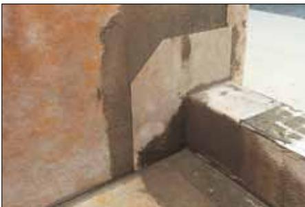
**14** Use KERDI-KERECK-F pre-formed inside and outside corners to seal the shower curb and/or bench to the walls and tray. The curb/tray and the bench/tray junctions are sealed using KERDI-BAND. Cover the curb and bench with KERDI.
