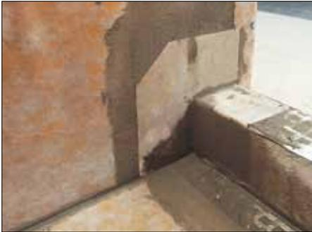
**8** Use KERDI-KERECK-F pre-formed inside and outside corners to seal the shower curb to the wall and mortar base. The curb/base junction is sealed using KERDI-BAND. Cover the curb with KERDI.
