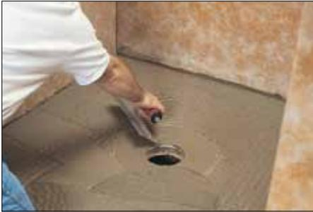
**9** If there is access to the plumbing from below and the waste line can be connected after installing the KERDI-DRAIN, apply unmodified thin-set mortar to the entire shower tray surface and completely fill the step in the shower tray.
