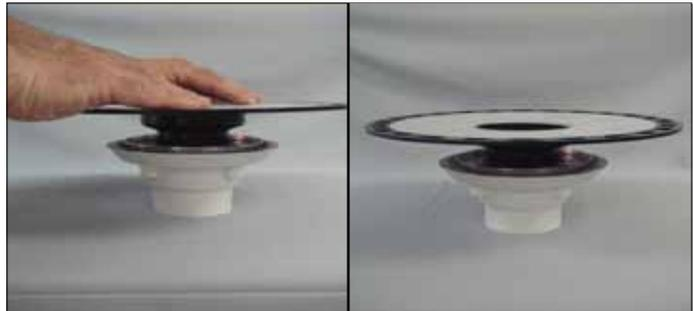
6 Slide adaptor flange into adaptor ring. Ensure full support under the adaptor flange with mortar or foam tray center section and thin-set mortar (not shown).
