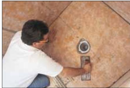
**12** Embed the KERDI waterproofing membrane into the mortar and work the matting onto the entire surface of the tray to ensure proper adhesion and to remove air pockets. Be sure the connection between the KERDI and KERDI-DRAIN is secure.
