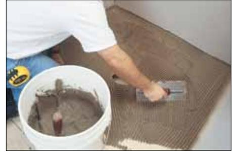
**2** Apply unmodified thin-set mortar to the substrate using a 1/4" x 3/8" (6 mm x 10 mm) square- or U-notched trowel. The floor must be level. Any leveling must be done prior to placing the tray.
