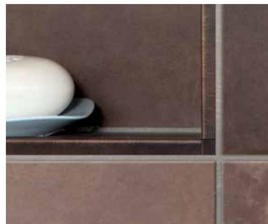
**QUADEC** square-shaped profile and corners applied to tile edges and outside corners of the shower including the shower bench and niche, and used to finish the tile base. **DILEX-AHK** cove-shaped profile and corners used to create a smooth transition between the walls and floor.
