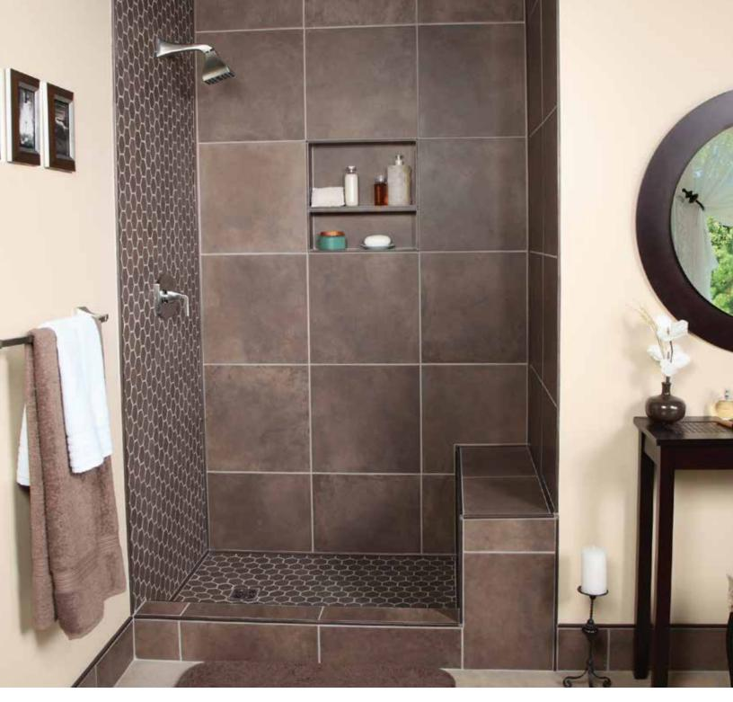
Hexagon shaped tiles installed on the floor and wall of this shower accent the design, while bronze profiles complement the rich brown colors and create clean finished edges and corners.
