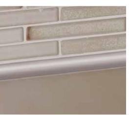
RONDEC-STEP edging profile applied to the sink rail. RONDEC bullnose profile and large radius sink corners used to produce the tiled-under sink. DILEX-AHK cove-shaped profile used to create a smooth transition between the countertop and backsplash.
