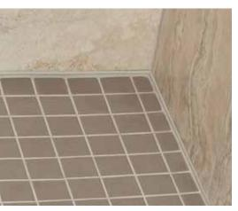
RONDEC bullnose profile used to finish the tile edges on the wall and tile base. DILEX-EKE PVC corner movement joint profile in classic grey used to create a seamless transition between the shower walls and floor.
