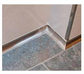
QUADEC square-shaped profile and corners applied to the tile edges of the bathtub skirting and wall tile, and used to trim the niches. QUADEC-FS double-rail edging profile applied to the sink rail. DILEX-EHK cove-shaped profile used to create smooth floor/wall and countertop/wall transitions.
