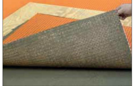
Lift up a corner of the matting to check coverage. Proper installation results in full contact between the fleece webbing and the thin-set mortar. Simply abut end and side sections of adjacent sheets.
