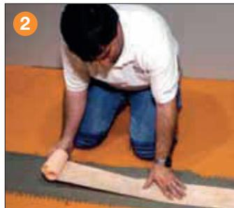
Comb additional unmodified thin-set mortar over the joint using a 1/4" x 3/16" (6 mm x 5 mm) V-notched trowel or the Schluter®-KERDI trowel, which features a 1/8" x 1/8" (3 mm x 3 mm) square-notched design. Using the flat side of the trowel, firmly press the 5" (127 mm)-wide Schluter®-KERDI-BAND into the mortar to ensure 100% coverage and to remove excess mortar and air pockets.
