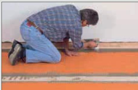
Today's construction methods, which include the use of lightweight, moisture-sensitive materials, such as plywood, OSB, and gypsum concrete, have made the installation of hard surface coverings particularly challenging. If wood or gypsum concrete substrates are exposed to moisture, the tile layer above can be damaged as a result.
