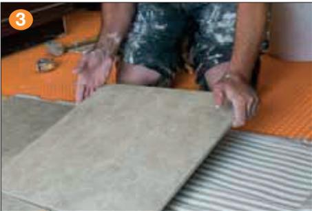
Tile can be installed over DITRA and DITRA-XL immediately; no need to wait for the mortar to cure. Fill the cut-back cavities with unmodified thin-set mortar and comb additional mortar over the matting using a trowel that is appropriate for the size of the tile. Solidly embed the tiles in the setting material. Periodically remove and check a tile to ensure that full coverage is being attained.
