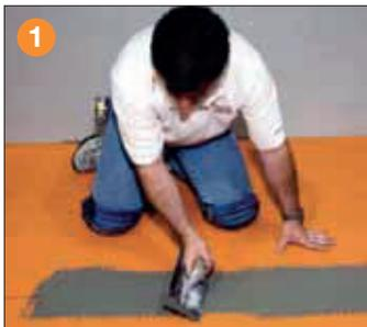
At the joints, fill the cut-back cavities with unmodified thin-set mortar, approximately 8" (203 mm) wide, centered over the joint.
