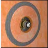
**8.1 Schluter®-KERDI-SEAL-MV** Mixing valve seal with over-molded rubber gasket
