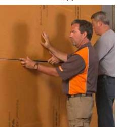
4 Use a level to check the wall to ensure it is now level, plumb, and flat to industry standards.
