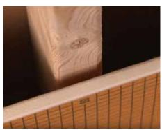
Mix thin-set mortar to be fairly stiff. Apply thin-set mortar to all applicable studs. Please note, thin-set mortar must be applied to the full stud (i.e., no spot bonding). Apply mortar more heavily on the bowed stud(s).
