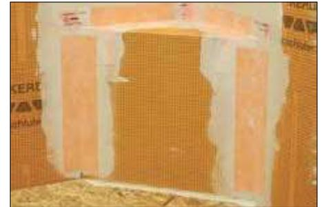
**3** Install KERDI-BAND and KERDI-KERECK and KERDI-KERS-B (for triangular bench) to cover all seams and corners, ensuring a minimum 2" (50 mm) overlap, and work the membrane into the mortar to achieve full coverage and remove air pockets.
