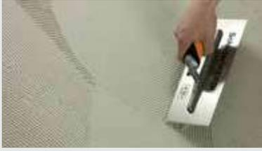
Schluter®-Systems offers thin-set mortars designed for use with Schluter® membranes and boards. All Schluter®-Systems' thin-set mortars, including the ALL-SET™ and FAST-SET™ modified varieties, can be used to set tile over Schluter®-DITRA, DITRA-HEAT, KERDI, KERDI-BOARD non absorptive substrates. If Schluter® thin-set mortars are not used, we require unmodified thin-set mortar when setting ceramic or porcelain tile over KERDI.
