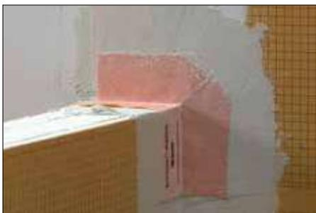
**7** Seal connections to knee walls using KERDI-KERECK-F preformed corners and Schluter SET™, ALL-SET™, FAST-SET™, or unmodified thin-set mortar.
