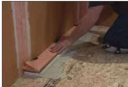
**2** Apply Schluter SET™, ALL-SET™, FAST-SET™, or unmodified thin-set mortar to the top of the channel support and press the channel body firmly into the mortar, ensuring full support of the bonding flange. Check to make sure the KERDI-LINE is level.
