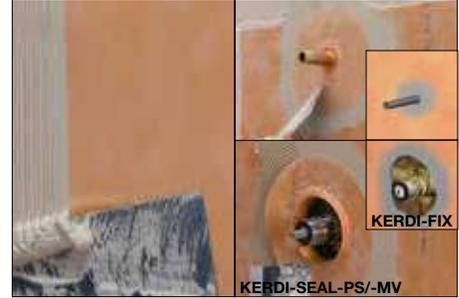
**3** Seams in the membrane are constructed by overlapping the edges by 2" (50 mm) or by abutting adjacent sheets and installing KERDI-BAND, centered over the joint. Any protrusions through the membrane (e.g., mixing valve, shower head, etc.) must be sealed with KERDI-SEAL-PS/-MV, KERDI-FIX, or other suitable sealant.
