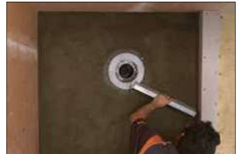
**2** The screed is then placed flush with the top of the bonding flange of the KERDI-DRAIN. Slope the mortar bed at 1/4" (6 mm) per 12" (305 mm) using the bonding flange and a perimeter screed as guides.
