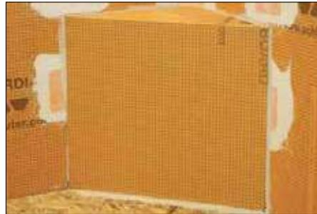
**2** Press the bench firmly into place and check the underside and backsides to ensure that full coverage and support are achieved. Verify that the slope on the surface of the bench is directed toward the shower base.
