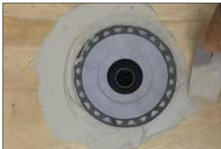
**2** Apply Schluter SET™, ALL-SET™, FAST-SET™, or unmodified thin-set mortar to the substrate and to the top and bottom of the detached center section of the KERDI-SHOWER-T/-TS/-TT tray. Slide the center section into place below the drain to ensure solid and uniform support of the bonding flange.
