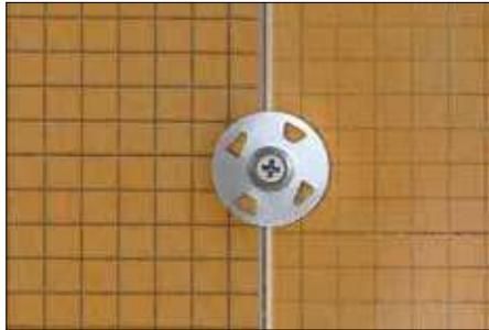
**2** Abut panels over the center of the studs or other solid backing. Screws may be placed between adjacent panels such that the washers fasten both panel edges. The maximum allowable on-center fastener spacing is 12" (30 cm) for walls and 6" (15 cm) for ceilings.
