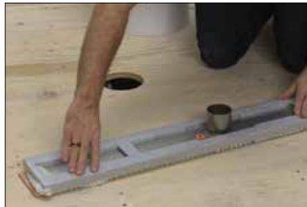
**2** Apply Schluter SET™, ALL-SET™, FAST-SET™, or unmodified thin-set mortar to the top of the channel support with a notched trowel and press the channel support firmly onto the underside of the channel body. Attach the mechanical coupling to the drain outlet and the cut section of the pipe per the coupling manufacturer's instructions.
