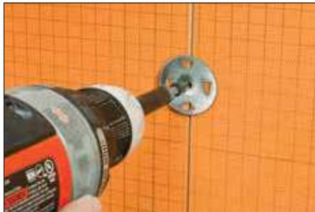
**2** Abut panels over the center of the studs. Screws may be placed between adjacent panels such that the washers fasten both panel edges. The maximum allowable on-center fastener spacing is 12" (30 cm) for walls and 6" (15 cm) for ceilings.
