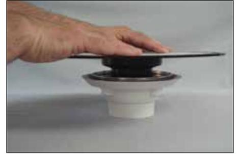
**3** Slide the adaptor flange into the adaptor ring and ensure full support underneath with mortar or the detachable center section of the foam tray. Depending on the installed drain elevation, it may be necessary to install a polystyrene foam panel, tile backerboard, etc. prior to the tray. Install the tray as per the instructions on page 22.
