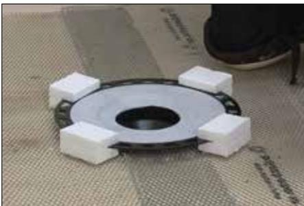
**1** Measure and cut a section of pipe to connect KERDI-DRAIN to the odor trap using the foam spacers included with the drain as a spacer. When installing KERDI-DRAIN over wood substrates, the minimum thickness of mortar required at the perimeter of the bonding flange is 1" (25 mm). Prepare the odor trap, cut section of pipe, and KERDI-DRAIN with cleaner, primer and ABS or PVC cement per the solvent cement manufacturer's instructions and connect.
