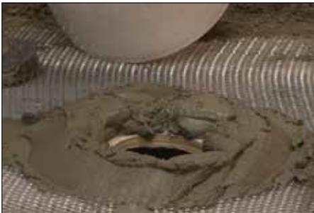
**1** Place a ring of loose mortar up to the inlet hole in the floor and firmly press the drain into the mortar and level. The bonding flange must be fully supported to prevent damage to the tile assembly (e.g., cracked grout around drain). When installing KERDI-DRAIN over wood substrates, the minimum thickness of mortar required at the perimeter of the bonding flange is 1" (25 mm).
