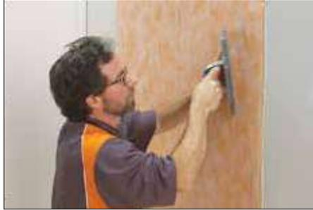
**2** Apply Schluter SET™, ALL-SET™, FAST-SET™, or unmodified thin-set mortar using a 1/4" x 3/16" (6 mm x 5 mm) V-notched trowel or the KERDI-TROWEL. Embed KERDI or KERDI-DS in the mortar and work the membrane onto the entire surface to ensure full coverage and remove air pockets.
