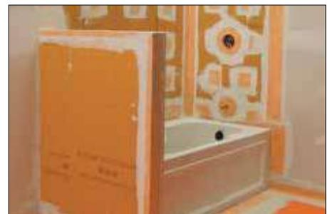
**8** Once all seams, corners, and knee walls have been completely sealed, the assembly is waterproofed and ready to be tiled.
