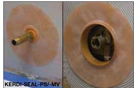
**6** Any protrusions through the panel (e.g., mixing valve, shower head, etc.) must be sealed with KERDI-SEAL-PS/-MV, KERDI-FIX, or other suitable sealant.
