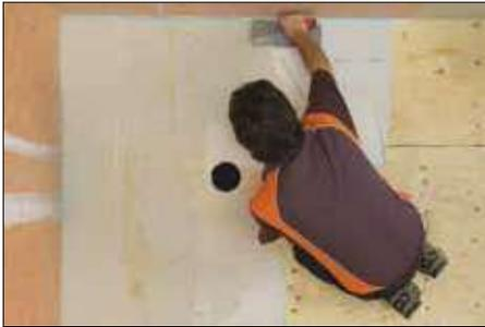
**1** Apply Schluter SET™, ALL-SET™, FAST-SET™, or unmodified thin-set mortar to the substrate using a 1/4" x 3/8" (6 mm x 10 mm) square- or U-notched trowel.
