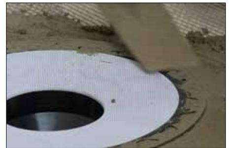
**2** Pack loose mortar under the drain up to the inlet hole to ensure solid and uniform support of the bonding flange and level. The mortar bed is then placed according to the instructions above.
