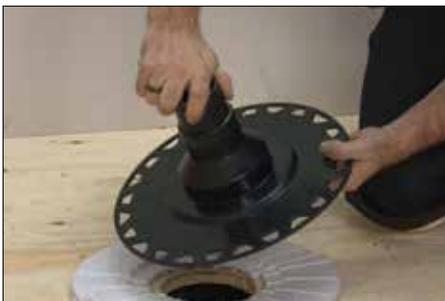
**1** Begin by dry-fitting the components. Measure and cut a section of pipe to connect KERDI-DRAIN to the odor trap using the detachable center section of the tray or foam spacers included with the drain as a spacer. Prepare the odor trap, pipe, and KERDI-DRAIN with cleaner, primer and ABS or PVC cement per the solvent cement manufacturer's instructions and connect.
