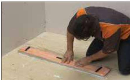
**4** Solidly embed the channel support and KERDI-LINE into the mortar on the floor and connect the cut section of pipe to the odor trap. Check to make sure the KERDI-LINE is level.
