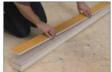
**Note:** Schluter®-KERDI-BOARD can be used to build custom curbs.
