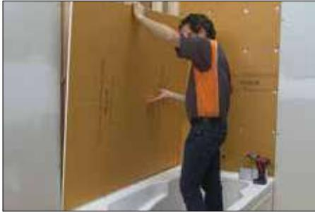
**1** KERDI-BOARD can be mounted vertically or horizontally on framing with appropriate screws (e.g., coarse thread wood screw for wood studs and self-tapping for metal studs) and corresponding KERDI-BOARD-ZT washers. Minimum board thickness = 1/2" (12.5 mm) for studs spaced at 16" (40.6 cm) o.c.; 3/4" (19 mm) for studs spaced at 24" (61.0 cm) o.c. Screws must reach a depth of at least 3/4" (20 mm) in wood studs and at least 3/8" (10 mm) in metal studs.
