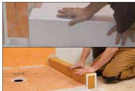
**2** Press the curb or ramp firmly into place. Check the underside of the curb or ramp to ensure that full coverage and support is achieved. **Note:** When setting tile on the curb, the surface must be sloped towards the shower drain.
