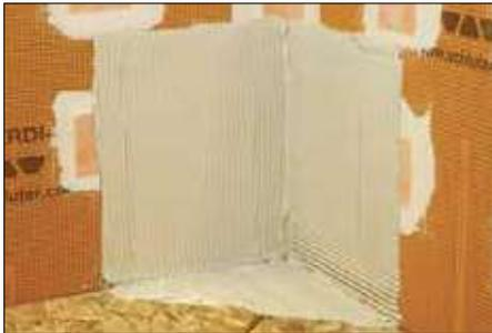
**1** Apply Schluter SET™, ALL-SET™, FAST-SET™, or unmodified thin-set mortar to the floor and walls using a 1/4" x 3/8" (6 mm x 10 mm) square- or U-notched trowel.
