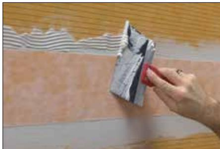
**5** KERDI-BOARD joints, corners, and fastener penetrations are sealed with KERDI-BAND, ensuring a minimum 2" (50 mm) overlap.
