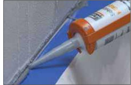
**3** Place painter's tape to protect the tub deck. Apply Schluter SET™, ALL-SET™, FAST-SET™, or unmodified thin-set mortar to the KERDI-BOARD using a 1/4" x 3/16" (6 mm x 5 mm) V-notched trowel or the KERDI-TROWEL. Completely fill the 1/4" (6 mm)-wide gap between the KERDI-BOARD and tub with KERDI-FIX or other suitable sealant.
