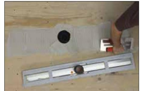
**3** Apply Schluter SET™, ALL-SET™, FAST-SET™, or unmodified thin-set mortar to the substrate where the drain is to be placed with a notched trowel. Prepare the cut section of pipe and odor trap with cleaner, primer and ABS or PVC cement per the solvent cement manufacturer's instructions.
