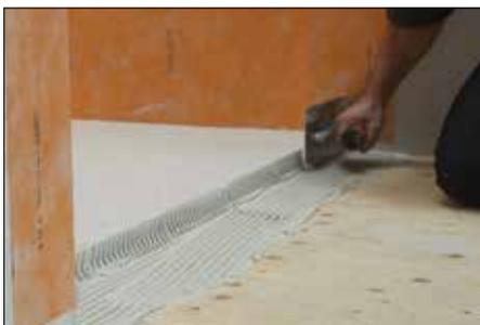
**1** Apply Schluter SET™, ALL-SET™, FAST-SET™, or unmodified thin-set mortar to the floor and to the edge of the shower base and walls using a 1/4" x 3/8" (6 mm x 10 mm) square- or U-notched trowel.
