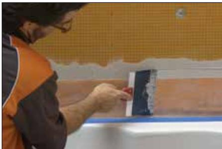
**4** Apply KERDI-BAND waterproofing strips. Solidly embed the membrane in the mortar and KERDI-FIX to ensure full coverage and remove air pockets.
