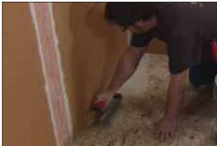
**1** Apply Schluter SET™, ALL-SET™, FAST-SET™, or unmodified thin-set mortar to the substrate where the drain is to be placed with a notched trowel and solidly embed the channel support in the mortar.
