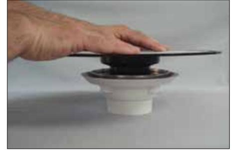
**3** Slide the adaptor flange into the adaptor ring and ensure full support under the adaptor flange with mortar. The mortar bed is then placed according to the instructions on page 23.
