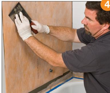
**4** Apply Schluter SET™, ALL-SET™, FAST-SET™, or unmodified thin-set mortar to the solid backing and previously applied KERDI-BAND. Embed the KERDI in the thin-set mortar and work the membrane onto the entire surface to ensure full coverage and remove air pockets.
