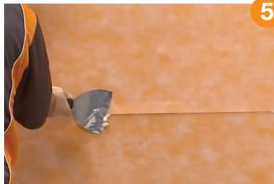
**5** Seams in the membrane are constructed by overlapping the edges of KERDI by 2" (50 mm).
