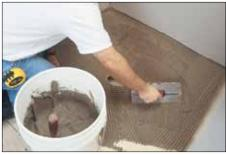
Apply unmodified thin-set mortar to the substrate using a 1/4" x 3/8" (6 mm x 10 mm) square- or U-notched trowel. The floor must be level. Any leveling must be done prior to placing the tray.
