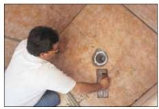
Embed the KERDI waterproofing membrane into the mortar and work the matting onto the entire surface of the tray to ensure proper adhesion and to remove air pockets. Be sure the connection between the KERDI and KERDI-DRAIN is secure.
