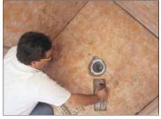
Apply the KERDI membrane to the entire surface of the mortar bed. The KERDI is carried to the step in the bonding flange (template provided). Be sure the connection between the KERDI and KERDI-DRAIN is secure.
