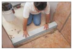
If necessary, cut the KERDI-SHOWER-SC curb to length using a handsaw. Apply unmodified thin-set mortar to the floor and to the edge of the shower tray and walls using a 1/4" x 3/8" (6 mm x 10 mm) square- or U-notched trowel, and press the curb firmly into place. Check the underside of the curb to ensure that full coverage and support is achieved.
