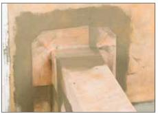
Seal connections to knee walls using KERDI-KERECK-F preformed outside corners and unmodified thin-set mortar.
