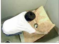
Apply unmodified thin-set mortar to the shower base. When using the ABS or PVC drain, apply additional unmodified thin-set mortar to the top of the fleece-laminated bonding flange. When using the stainless steel drain, KERDI is adhered to the bonding flange with the KERDI-FIX adhesive/sealant. The stainless steel bonding flange must be clean and free of grease or other contaminants prior to KERDI-FIX application.
