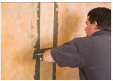
Seams are constructed by overlapping the edges of KERDI by a minimum of 2" (50 mm) or by butting adjacent sheets of KERDI and installing KERDI-BAND with unmodified thin-set mortar, centered over the joint.
