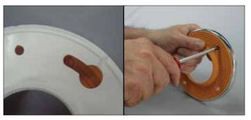
Align the bolt pattern of the clamping ring with the matching punchouts in the adaptor ring. Punch the matching inserts out through the stainless steel adaptor ring.
