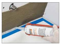
Place painter's tape to protect the tub deck. Construct tub/wall connections using the KERDI-BAND waterproofing strip or 5" (125 mm)-wide cut sections of KERDI water-proofing membrane. Apply unmodified thin-set mortar to solid backing and completely fill the 1/4" (6 mm)-wide gap between the solid backing and tub with KERDI-FIX or an equivalent sealant.
