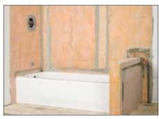
The KERDI waterproofing application is now complete. Using a trowel that is appropriate for the size of the tile, apply unmodified thin-set mortar directly to the exposed KERDI surface and install the tiles, ensuring full coverage.
