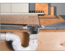
The grate assembly is installed in conjunction with the tile. Place the height adjustment collar inside the lateral adjustment ring and snap the grate into place. Fill the step in the bonding flange with thin-set mortar and back-butter the underside of the grate to ensure full support. Press the assembly into the mortar and install the surrounding tiles. Position the grate to match the joint pattern of the tile covering and press flush with the tile surface.
