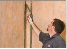
Install KERDI-BAND at inside wall corners and wall/ceiling junctions\* using unmodified thinset mortar, centered over the joints. Install KERDI-KERECK-F pre-formed corners at inside
