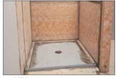
OPTION: Walls can be waterproofed Schluter®-KERDI prior to the installation of tray. Floor/wall connections are constructed with Schluter®-KERDI-BAND after installing the tray.
