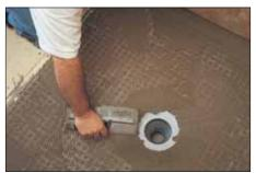
When using the ABS or PVC drain, apply additional unmodified thin-set mortar to the top of the fleece-laminated bonding flange. When using the stainless steel drain, KERDI is adhered to the bonding flange with the KERDI-FIX adhesive/sealant. The stainless steel bonding flange must be clean and free of grease or other contaminants prior to KERDI-FIX application.
