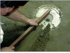
Fill the remainder of the shower base with Slope the mortar bed using the mortar. bonding flange and the perimeter screed as a screeding guide. As soon as the mortar bed can be walked upon, waterproofing with the KERDI membrane can begin.
