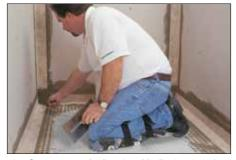
Construct tray/wall and wall/ceiling\* connections and seal vertical inside corners using the KERDI-BAND waterproofing strip or 5" (125 mm)-wide cut sections of KERDI waterproofing membrane. Install KERDI-KERECK-F pre-formed corners at inside corners.
