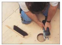
After locating the correct position for the drain, cut a hole in the substrate using the template provided. Note: A larger hole can lead to lack of support and damage to the tile assembly (e.g., cracked grout around the drain).
