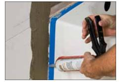
Protect walls and ceiling\* from moisture and vapor penetration using KERDI. Apply unmodified thin-set mortar to walls and completely fill the 1/4" (6 mm)-wide gap between the solid backing and tub with KERDI-FIX or an equivalent sealant.
