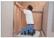
Protect walls and ceiling\* from moisture and vapor penetration using KERDI. Seams are constructed by overlapping the edges of KERDI by 2" (50 mm) minimum or by butting adjacent sheets of KERDI and installing KERDI-BAND, centered over the joint.
