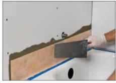
Solidly embed KERDI-BAND in the mortar and KERĎI-FIX.
