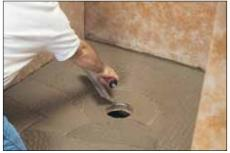
If there is access to the plumbing from below and the waste line can be connected after installing the KERDI-DRAIN, apply unmodified thin-set mortar to the entire shower tray surface and completely fill the step in the shower tray.
