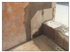
Use KERDI-KERECK-F pre-formed inside and outside corners to seal the shower curb to the wall and mortar base. The curb/base junction is sealed using KERDI-BAND. Cover the curb
