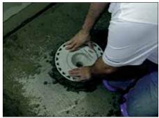
Place a ring of loose mortar up to the inlet hole in the floor and firmly press the drain into the mortar. The bonding flange must be fully supported to prevent damage to the tile assembly (e.g., cracked grout around drain).
