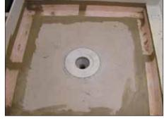
Construct floor/wall and wall/ceiling\* connections and seal vertical inside corners using the KERDI-BAND waterproofing strip or 5" (125 mm)-wide cut sections of KERDI waterproofing membrane. Install KERDI-KERECK-F pre-formed corners at inside corners.
