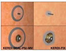
Install KERDI-SEAL-PS pipe seals at showerhead, body sprays, etc. and KERDI-SEAL-MV mixing valve seal at the mixing valve. As an alternative, KERDI-FIX or equivalent sealant can be used to seal pipe protrusions and protect moisture-sensitive solid backing panels at the mixing valve.
