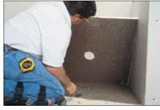
Check the underside of the tray to ensure that full coverage and support are achieved.
