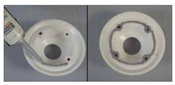
Apply a continuous 1/4" - 3/8" (6 mm - 10 mm) bead of Schluter®-KERDI-FIX to the installed drain flange.
