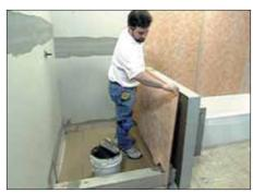
Protect walls and ceiling\* from moisture and vapor penetration using KERDI. Seams are constructed by overlapping the edges of KERDI by 2" (50 mm) minimum or by butting adjacent sheets of KERDI and installing KERDI-BAND, centered over the joint.
