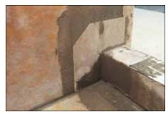
Use KERDI-KERECK-F pre-formed inside and outside corners to seal the shower curb and/ or bench to the walls and tray. The curb/tray and the bench/tray junctions are sealed using KERDI-BAND. Cover the curb and bench with KERDI.
