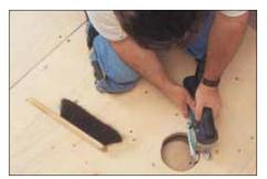
After locating the correct position for the drain, cut a hole in the substrate using KERDI-SHOWER-ST tray as a template. Note: A larger hole can lead to lack of support and damage the tile assembly (e.g., cracked grout around drain).
