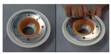
Align the holes in the adaptor ring with the bolt holes in the installed drain and place the adaptor ring on the installed drain flange. Re-insert bolts.
