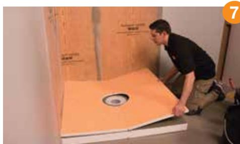
Apply Schluter SET®, ALL-SET®, FAST-SET®, or unmodified thin-set mortar to the top of the KERDI-SHOWER-CB compensation board using a 1/4" x 3/8" (6 mm x 10 mm) square- or U-notched trowel. Place the KERDI-SHOWER tray and solidly embed in the mortar.
