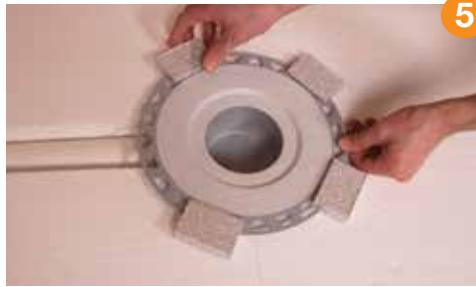
Dry fit the plumbing components. Measure and cut a section of pipe to connect KERDI-DRAIN-H to the odor trap using the detachable center section of the tray, or foam spacers included with the drain, as a spacer. Proper slope MUST be maintained to ensure adequate drainage. Prepare the pipe and KERDI-DRAIN-H with cleaner, primer, and ABS or PVC cement per the solvent cement manufacturer's installation instructions and connect.
