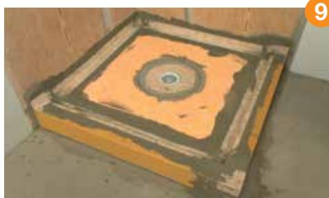
Seal inside corners by abutting adjacent sheets and installing KERDI-BAND with Schluter SET®, ALL-SET®, FAST-SET®, or unmodified thin-set mortar, centered over the joint. Install KERDI-KERECK prefabricated waterproofing corners at all inside and outside corners. When using the KERDI-BOARD-SC curb, seal the curb to the base and walls using KERDI-KERECK and KERDI-BAND.
