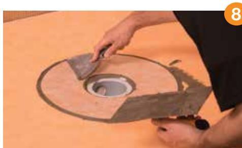
Apply Schluter SET®, ALL-SET®, FAST-SET®, or unmodified thin-set mortar to the bonding flange and recess area in the tray with a 1/4" x 3/16" (6 mm x 5 mm) V-notched trowel or the KERDI-TROWEL. The thin-set mortar must be mixed to a fairly fluid consistency, but still able to hold a notch. Embed the KERDI membrane collar in the bond coat and work the membrane onto the KERDI-DRAIN bonding flange and shower base to ensure full coverage and remove air pockets.
