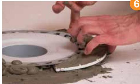
Apply Schluter SET®, ALL-SET®, FAST-SET®, or unmodified thin-set mortar to the KERDI-SHOWER-CB compensation board and to the top and bottom of the detached center section of the KERDI-SHOWER tray. Slide the center section into place below the drain to ensure solid and uniform support of the bonding flange.
