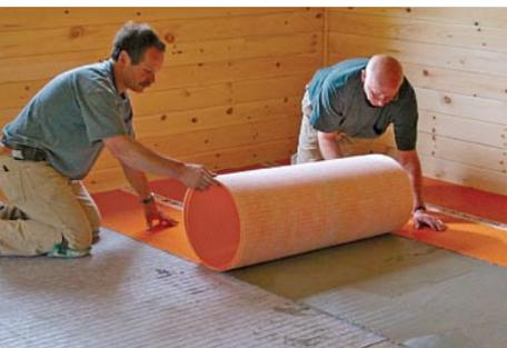
**One course at a time.** Spread only enough mortar for one course of membrane, then roll out the precut pieces.
