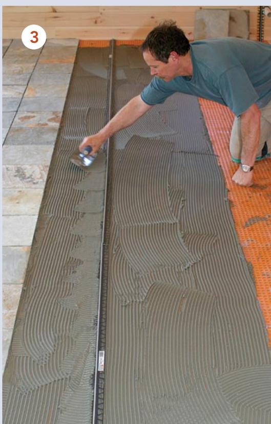
two layout lines intersect (photo top right). As I work down the floor, I apply thinset to an area in which I can set tile within about 15 minutes, usually about 30 sq. ft. at a time. For each set of courses, I install the first tile at the intersection of the layout lines. As each tile goes in, I apply a little downward pressure and slide the tile into place, which helps to lock the tile into the layer of thinset.
