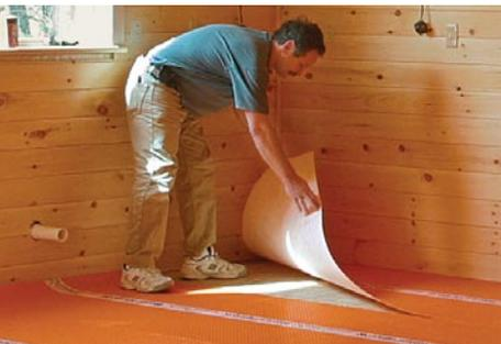
**Test-fit first.** Cut membrane to fit the floor with scissors or a utility knife. Cover the subfloor completely.
