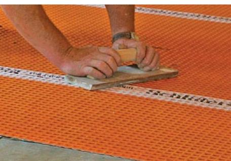
**Make a good impression.** After the membrane is rolled out flat, a wooden float ensures a good bond with the mortar.
