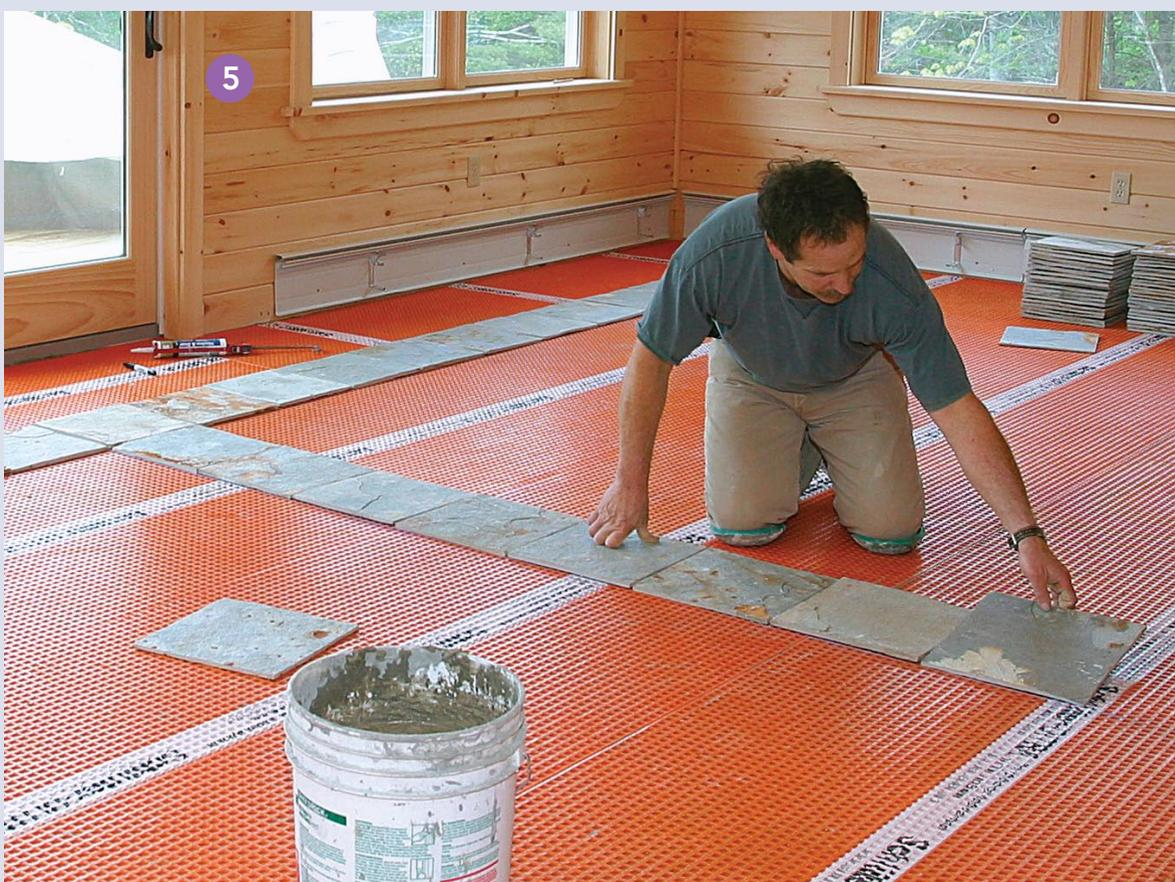
found that centering the tile on the middle of the door left 11-in. pieces on both sides of the room for minimal waste. Before lifting the tiles in front of the door, I marked the center tile's edge.
