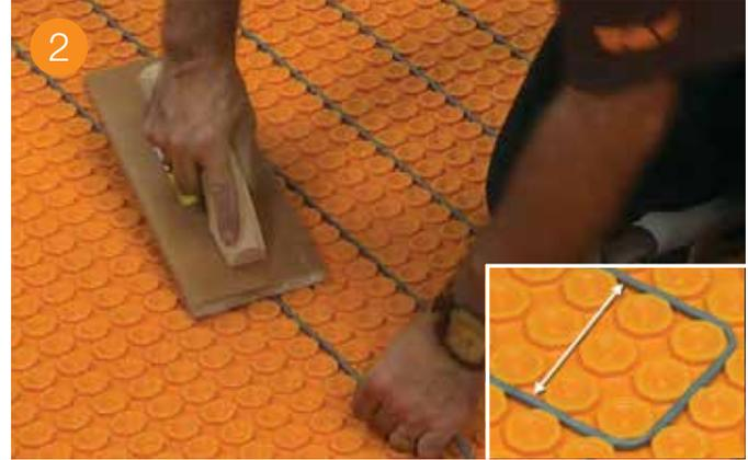
Embed the heating cables between studs, at a spacing of 3 studs or at a continuously alternating 3 stud - 2 stud sequence, depending on your application. For details, see the Ditra-Heat Installation Handbook in the Floor Warming section at [www.schluter.com](http://www.schluter.com) or [www.schluter.ca](http://www.schluter.ca)
