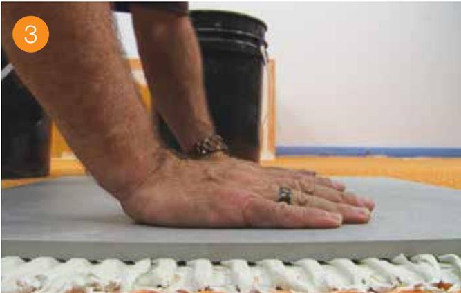
Using Schluter SET™, ALL-SET™, FAST-SET™, or unmodified thin-set mortar, tile can be installed over DITRA-HEAT and DITRA-HEAT-DUO immediately; no need for self-levelers.
