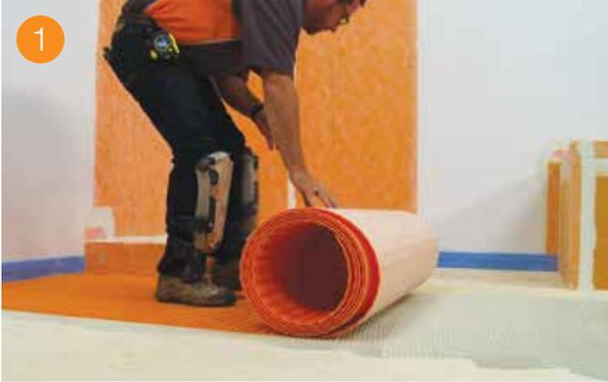
Using a thin set mortar appropriate for your sub-floor, apply DITRA-HEAT or DITRA-HEAT-DUO to the floor, fleece side down.
