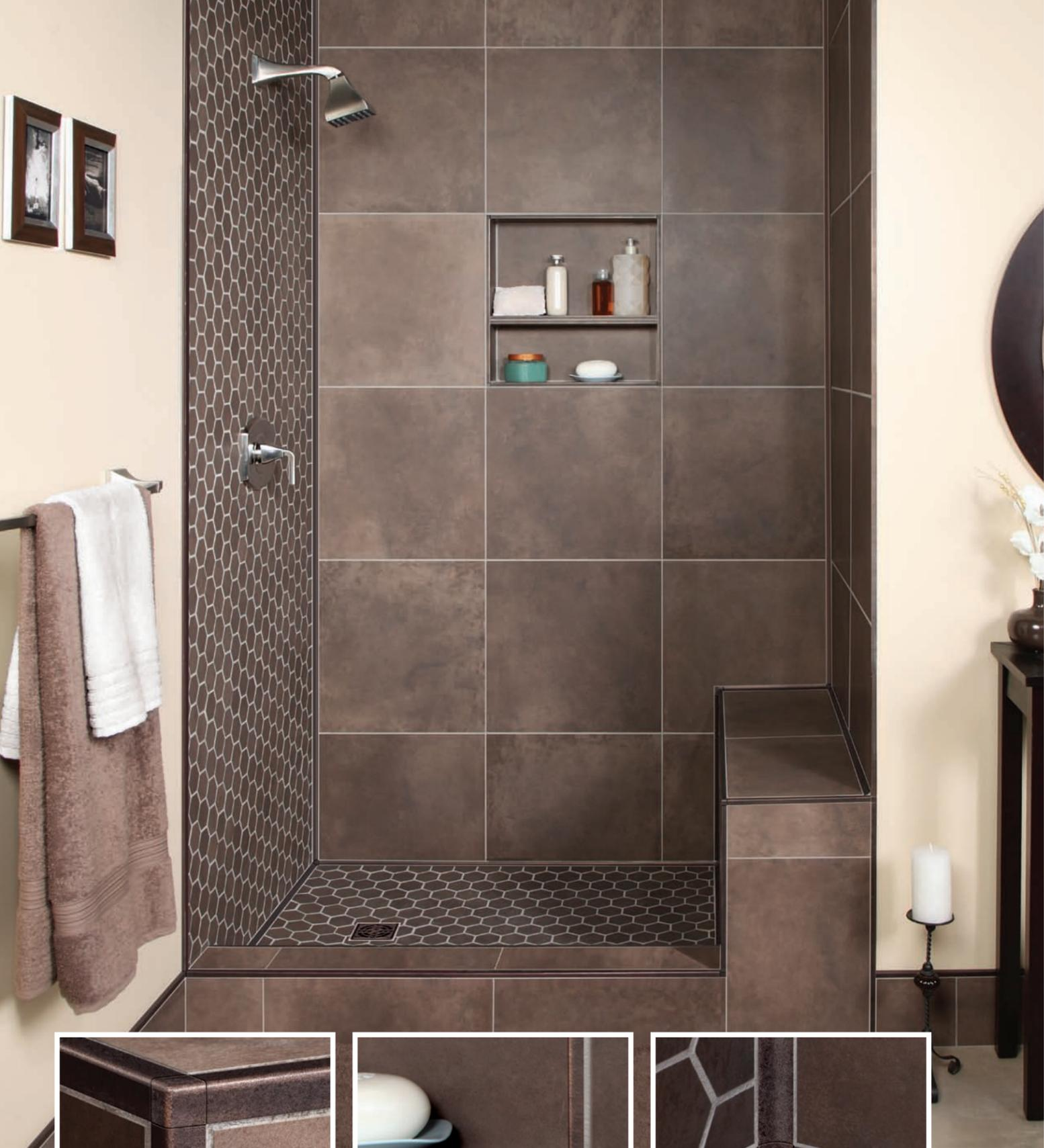
Schluter®-QUADEC edging profile and corners in Tuscan bronze applied to tile edges and outside corners of the shower including the shower bench and niche, and used to finish the tile base. Schluter®-DILEX-AHK cove-shaped profile and corners in Tuscan bronze used to create a smooth transition between the walls and floor.
