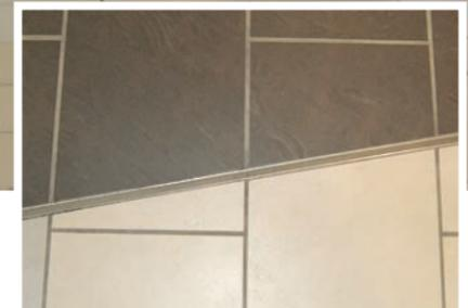
*Schluter®-DITRA uncoupling membrane installed over the concrete slab allowed the Schluter®-DILEX-KSN movement joint profile to be placed along one of the curves to create a natural-looking break between the two different tile colors.*
