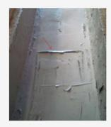
If applying over an existing coating: When over-coating existing coatings, compatibility and adhesion testing is recommended, and existing coating must be acknowledged as determining the adhesion and performance of all subsequently applied materials. When over-coating an existing coating, the entire surface must be sanded to remove all gloss. If an old coating is not sanded properly, this can result in peeling due to lack of adhesion.
