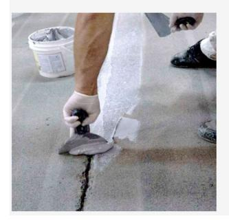
Any cracks or holes should be repaired using a crack filler prior to epoxy application. The CTM Epoxy Garage kit is **NOT** to be used to fill cracks or holes. Be sure to follow the instructions from the crack filler chosen.
