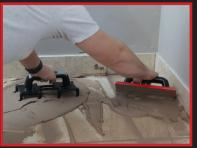
Ideal for troweling mortar on large format and GPTP installations
