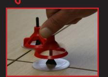
Easily spin the Leveling Cap down to the tile surface
