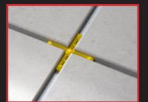
Leave-in grout joint & grout over
