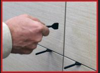
Breakaway post can be used as spacer or wall shims
