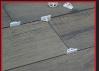
Ensures straight grout lines in any offset tile installation
