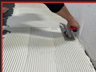
Low profile handle for proper angle in tighter spaces
