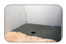
Step 2: ADHERE PROVA PAN® TO SUBSTRATE
