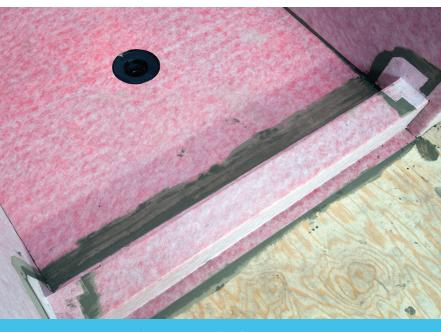
1. Dry fit the PROVA PAN<sup>®</sup> or PROVA PAN-MULTI<sup>®</sup> and PROVA DRAIN<sup>®</sup> to make sure drain pipe is at correct height for proper installation. The top of the drain pipe should measure between 1-3/8" to 1-5/8" below top of substrate.
