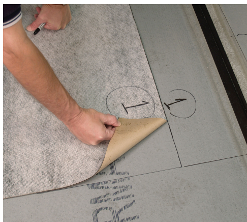
Measure and cut into sheets.
