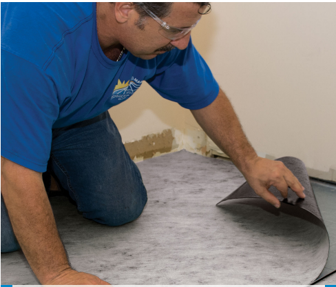
Remove the liner and apply down over the primed substrate.
