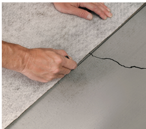
Dry-fit in place.
