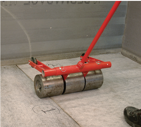
Ensure proper bond using a roller.
