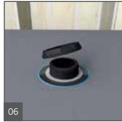
Tighten the gaskets firmly to the bases' steel ring using the locking nut. Make sure the drain body is still safely received in the valve-bead of sealant. Smooth out excess sealant over the drain body's flange surface.
