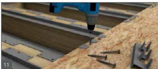
Use the flat head Phillips self-drilling screws with wings provided by wedi to fasten C brackets to the edge of the wood floor plate at the open side of the shower area. Fit the brackets between flanges of the joist/wall brackets. Use two screws to fasten this bracket through the wood floor and into the lower claws. When working with floor joists with a spacing greater than 16 in., use one full C bracket, and another one cut to length for full support along the edge of the floor.
