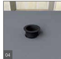
Drop the drain body firmly into the sealant.
