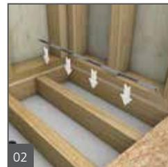
02 Cut the joist brackets to the length of the exposed floor joists. Depending on length and direction of floor joists, you may need to add a shorter joist bracket. Do not use joist brackets shorter than 12 in. (304.8 mm), or equipped with less than two (at least partial) mounting flanges.
