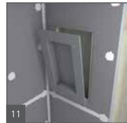
2 Fasteners on each side of the niche are set to create a flush transition to the wall panels. Another 1/2" (12.7 mm) bead of wedi sealant is spread over fasteners and seams.
