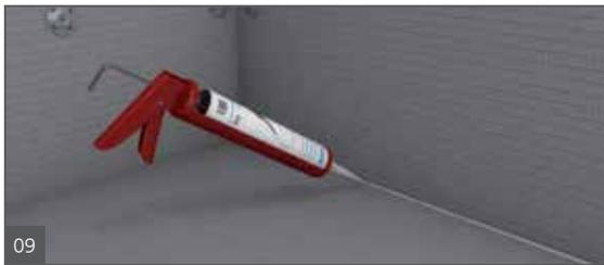
Apply a continuous 1/2" (12.7 mm) bead of sealant between all connections of panels and install with tightly butted seams. Excess sealant must be spread flat with a putty knife. All seams and fastener heads in the assembly are covered with a secondary 1/2" (12.7 mm) bead of sealant and spread flat. The seams should be covered 1" (25.4 mm) on either side of seam. All fastener/washers are covered with sealant stretching 1" (25.4 mm) over the washer edges.
