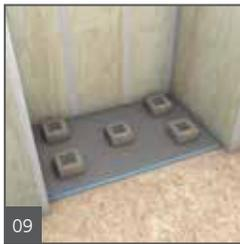
Press the Fundo firmly into the thinset bed, ensuring that the installation is level and void free. Apply some weight equally and leave on surface and drain area to allow the thinset to initially cure without being disturbed (e.g. thinset bags).
