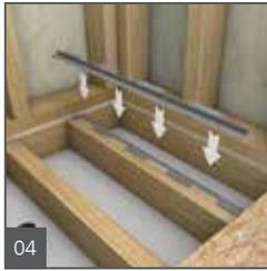
Fasten the next bracket on the other side of the floor joist. The mounting tabs must be staggered from those on the first bracket; this may require cutting the second bracket.
