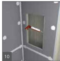
wedi Niches are installed in a cut out in the wedi wall and attached with its flange right into the center of 16" (406.4 mm) o.c. studs. wedi Joint Sealant is set along the connection of wall to niche.
