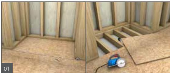
01 Measure and mark the area of subfloor to be removed. Use a circular saw to cut close to the framing. wedi recommends a combination of saws (i.e. sawzall or rotary cutter tool) where a standard circular saw might not reach.
