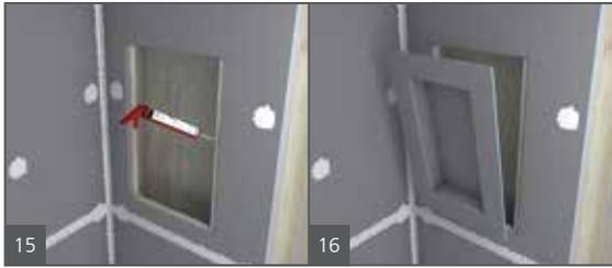
wedi Niches are installed in a cut out in the wedi wall and attached with it's flange right into the center of 16" (406.4 mm) o.c. studs. wedi Joint Sealant is set along the connection of wall to niche.
