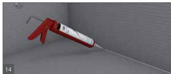
Apply continuous 1/2" (12.7 mm) beads of sealant between all connections of panels and install with tightly butted seams. Excess sealant must be spread flat with a putty knife. All seams and fastener heads in the assembly are covered with a secondary 1/2" (12.7 mm) bead of sealant and spread flat. The seams should be covered 1" (25.4 mm) on either side of seam. All fastener/washers are covered with sealant stretching 1" (25.4 mm) over the washer edges.
