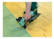
Continue laying the floor across the room. Lay the boards at an angle about 30° along the longer edge.
