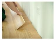
During the installation use a tapping block and a hammer to fit in the boards together along the longer edge. Adjust the tapping block along the entire longer edge of the board and tap it with hammer.
