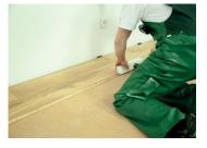
Fit the last board against the wall by tapping it with parquet shunting tool. Remember to leave an expansion gap of at least 3/8" (9.5 mm).
