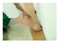
the glue manufacturer. Glue should be distributed over a maximum of two rows of boards. The interval between applying the glue and laying the boards should not exceed 40 minutes. When fitting boards using expansion wedges, use expansion gaps at least 3/8" (9.5 mm) wide. An expansion gap should be made along the perimeter of the room and around any other obstructions. Start the installation at the left side of the wall and continue towards the right side.
