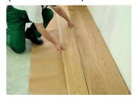
When fitting boards using expansion wedges, use expansion gaps at least 3/8" (9.5 mm) wide. An expansion gap should be made along the perimeter of the room and around any other ob-structions. Start the installation at the left side of the wall and continue towards the right side.
