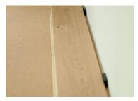
Fit in another board next to the first board. The boards should touch each other along the shorter edge. Begin the second row, starting with the off-cut from the first row. The recom- mended minimum length for the board starting the next floor row is 11.8" (300 mm). The recommended offset of connections between the boards along the shorter edge is 19.6" (500 mm). Continue laying the floor across the room.
