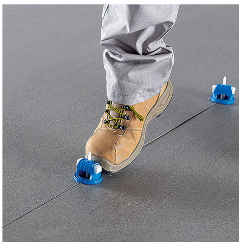
MapeLevel EasyClick Cap removal, showing the release of the spacer fragment
