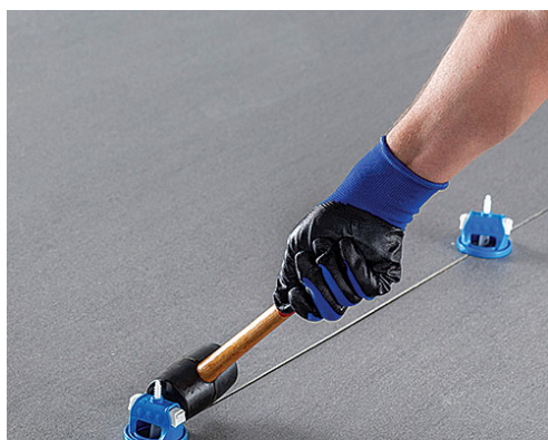
MapeLevel EasyClick Cap removal, showing the release of the spacer fragment
