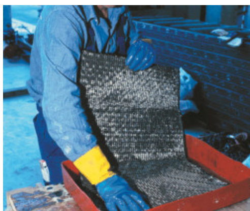
Manually impregnating MapeWrap C
