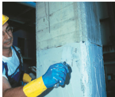
Smoothing with MapeWrap 11 or MapeWrap 12
