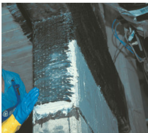
Wrapping columns and beams
