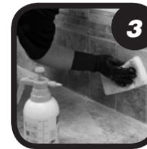
**Step 1:** Using the white nylon scrub pad, lightly scrub the grouted surface in a circular pattern over the surface. Also pass the scrub pad lightly over the joint to work the grout down to the desired height level and smoothness. This is the most critical stage for loosening the epoxy from the surface (Figure 4).
