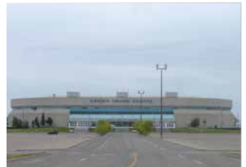
Sasktel Centre Saskatoon, Saskatchewan
