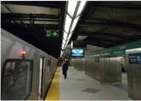
Toronto Transit Commission Subway
