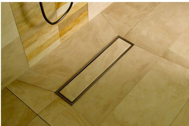
Linear drain—cover filled with tile.
