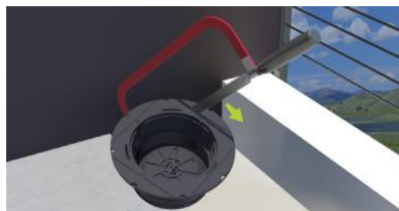
1. Cut one side of the pedestal.
