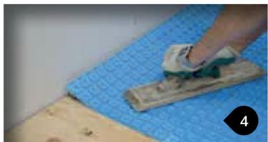
Unroll the membrane onto the thinset mortar and apply uniform pressure with a wood trowel.
