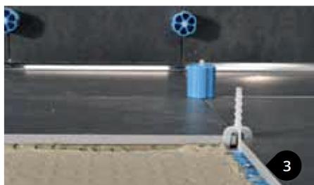
Carefully lay the tiles and press them on the layer of mortar. If a layer of skin has formed on the mortar, remove and apply again.
