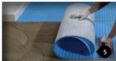
Lay the next sheet of the membrane, taking care to align it with the previous one, without overlapping. Align the square studs to facilitate the installation of the heating cables.
