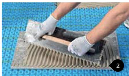
Apply the mortar to the back of the tiles with a notched trowel and lay them on the layer of mortar previously applied. Occasionally remove and check some tiles, to ensure full back coverage.
