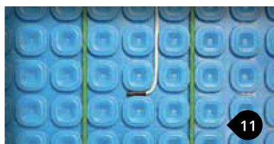
Install the floor sensor between 2 cable runs.
