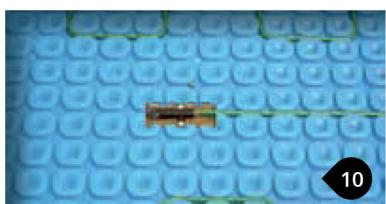
Finish the cable's installation by cutting the membrane and inserting the end of the cable.
