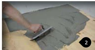
Key in the appropriate thinset mortar to the subfloor using the flat side of a trowel.
