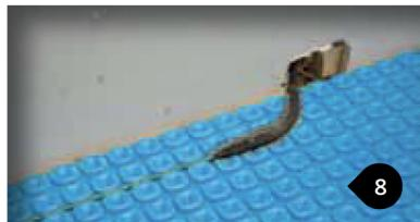
Start the installation of FLEXDECO's Cable by cutting the membrane to insert the mechanical joint and part of the cold lead.
