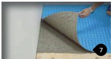
Check the thinset mortar transfer to the membrane. In case of partial coverage, increase the amount of adhesive or its fluidity.
