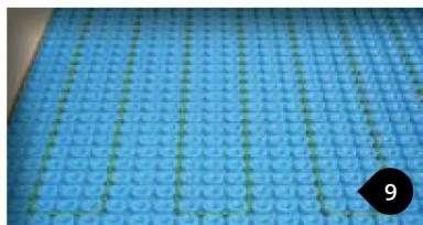
Insert the cable according to the installation guide, making sure to install the cable evenly at every 3 studs for a maximum output of 11.5W/ft<sup>2</sup>.
