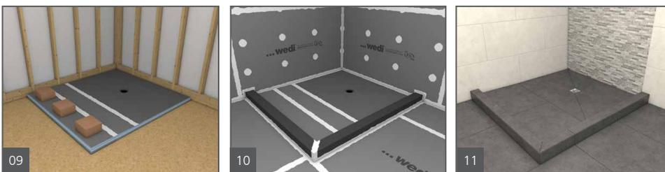
9. Weights are applied equally over the shower floor to promote a firmer bond with the thinset mortar allowing you to continue working on the shower walls immediately.
