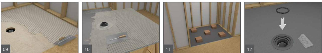
9. Clean the subfloor with a moist sponge to remove dust and dirt, and apply a skimcoat of a suitable, modified tile adhesive/ thinset (ANSI 118.4 or better), and comb through with a 1/4 in. x 1/4 in. notched trowel. Notches should be applied uniformly and point towards the shortest side of the base area. You can also use a 1/2 in. square notch trowel, instead.
