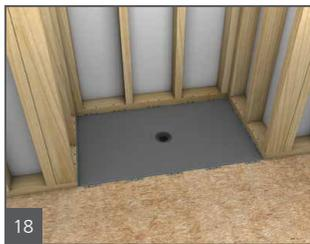
17. Install the wedi Fundo Ligno shower base in a bed of tile adhesive as per the Ligno installation manual.
