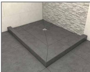
17. Option 2: The installation can now be completed using wedi Building Panel for walls and wedi curbs to separate the sloped shower floor from the flat bathroom floor.
