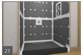
25. Weight is applied for a minimum of 30 minutes on and against the curb (from outside) and another 1/2 in. bead of sealant is applied over all curb seams and spread flat. The seams must be covered 1 in. either side of a seam.
