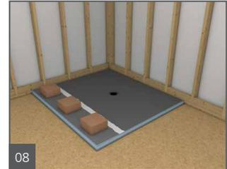
5. Apply a modified thinset bed on the subfloor as well as on the underside of the extension using a 1/4 in. x 1/4 in. square notch trowel on each surface. Make sure the mortar does not contaminate the joint sealant.
