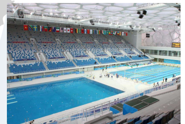
Beijing National Aquatics Centre | Beijing, China
