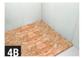
Install one of the recommended underlayment substrates below directly on top of BARRICADE Thermal Shield.
