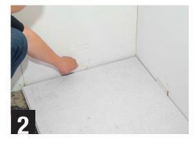
Start with a full panel with the grooved edges against the finished walls. Leave a 1/4" of space (for expansion) on rooms less than 20' long, and 1/2" for rooms longer than 20'.
