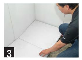
Install the first row of panels until you reach the end of that row, trimming the last panel to fit. If the resulting cut-off is greater than 18" long, you can use it to start the next run of panels. Some installers prefer taping the joints of the panels with a vapor barrier rated tape to help hold the panels in the first 1-2 rows together during installation.
