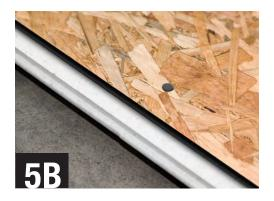
Screw down each panel of OSB, plywood or any other substrate used. Depending on the thickness of the substrate chosen, screws must penetrate the concrete a minimum 3/4". BARRICADE Thermal Shield is 1" in thickness, therefore, a 3/8" substrate would require a nail no shorter than 2 1/4" in length.
