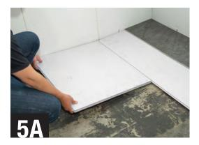
Work your way across the room installing one row at a time of the BARRICADE Thermal Shield panels, then the finished floor treatment, until the room is complete. Remember to stagger the joints of the BARRICADE Thermal Shield panels sufficiently row to row. Also, always follow the installation instructions of the finished floor as recommended by the manufacturer. Pay attention to acclimation requirements, and spacing at the room perimeter for expansion.
