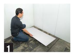
While you can lay the BARRICADE Thermal Shield panels in either direction, it is generally laid with the 4' length running the longest dimension of the room.
