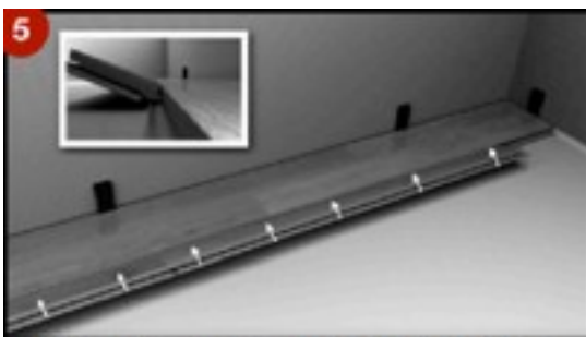
STEP 5: Keep the short side latches pushed parallel into the floor until tongue into groove
