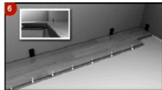
STEP 6: Make sure that the long side and short side tongue into the groove, and then drop down 2 pieces floor
