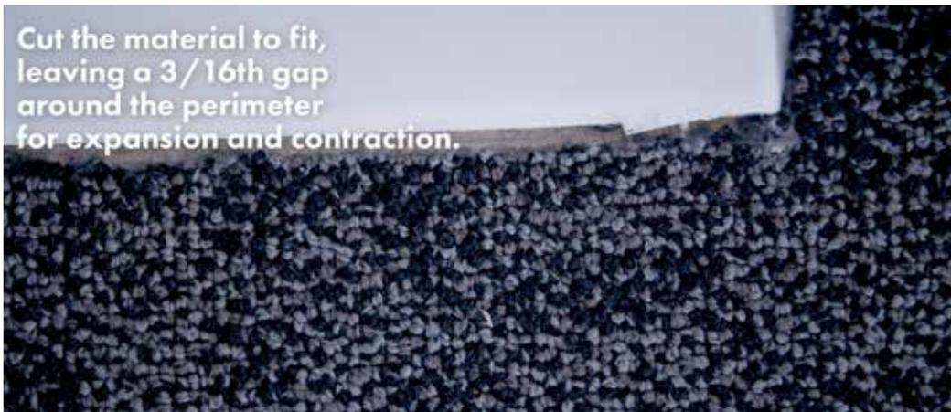
5. Pre-cut the seams of the PermaFuseXL using a utility knife with a new blade for each seam and a straight edge to ensure a perfect edge to seam together.
