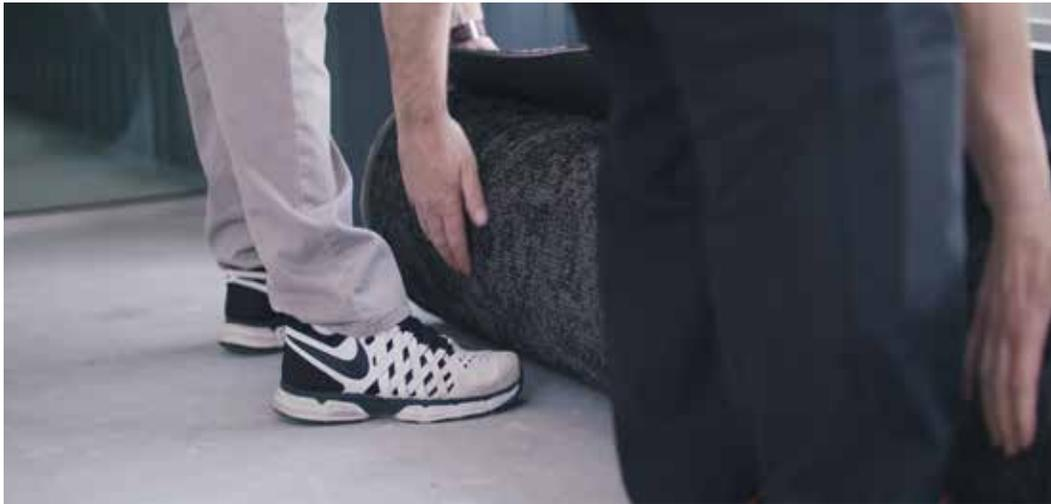
2. Ensure the substrate you are floating over is clean and free of debris, lumps, bumps and holes to ensure a flawless installation.
