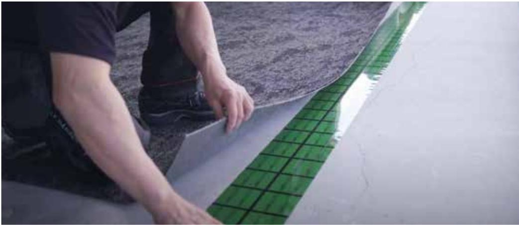
7. Fold back the PermaFuseXL at each seam location, remove the liner of the FuseMax seaming tape and place the tape under the seam sticky side up.
